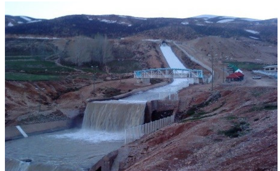
Fig. 2. Koohrang Tunnel in the Winter.
