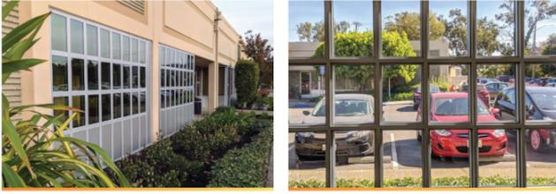
**Fig. 4.** A ubiquitous energy transparent photovoltaic window was installed in Redwood, California, as a field demonstration [37].
